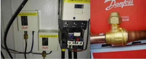
Use Danfoss world's number one brand for expansion valve, switches including high pressure protection and low pressure protection switch.
