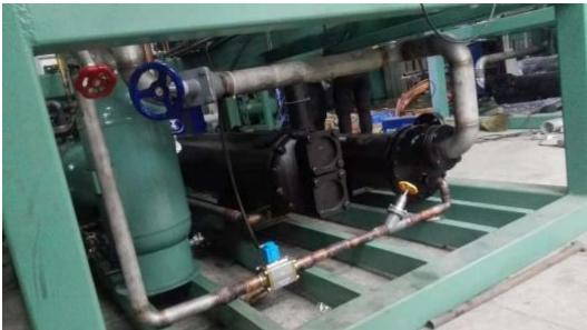
Maintenance is simplified with shut-off valves strategically placed at both ends of each accessory pipeline.
