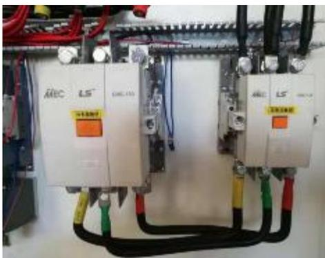
LG Brand Contactors, Air Switches
