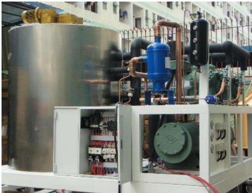
Refrigeration pipelines use high-quality copper tubes to AS/NZS1571 standard and we use 15% silver solder from us supplier Lincoln Electric.
