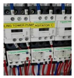
Schneider UL Electrical Contactors
